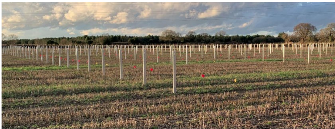
Figure 15.11 Mounting Structure Piles being Installed (taken at Tiln Farm, Retford, in January 2023)
